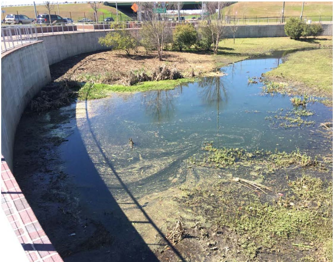
Figure 10 Fairview Environmental Park out-flow. Photo taken March 3, 2017.
