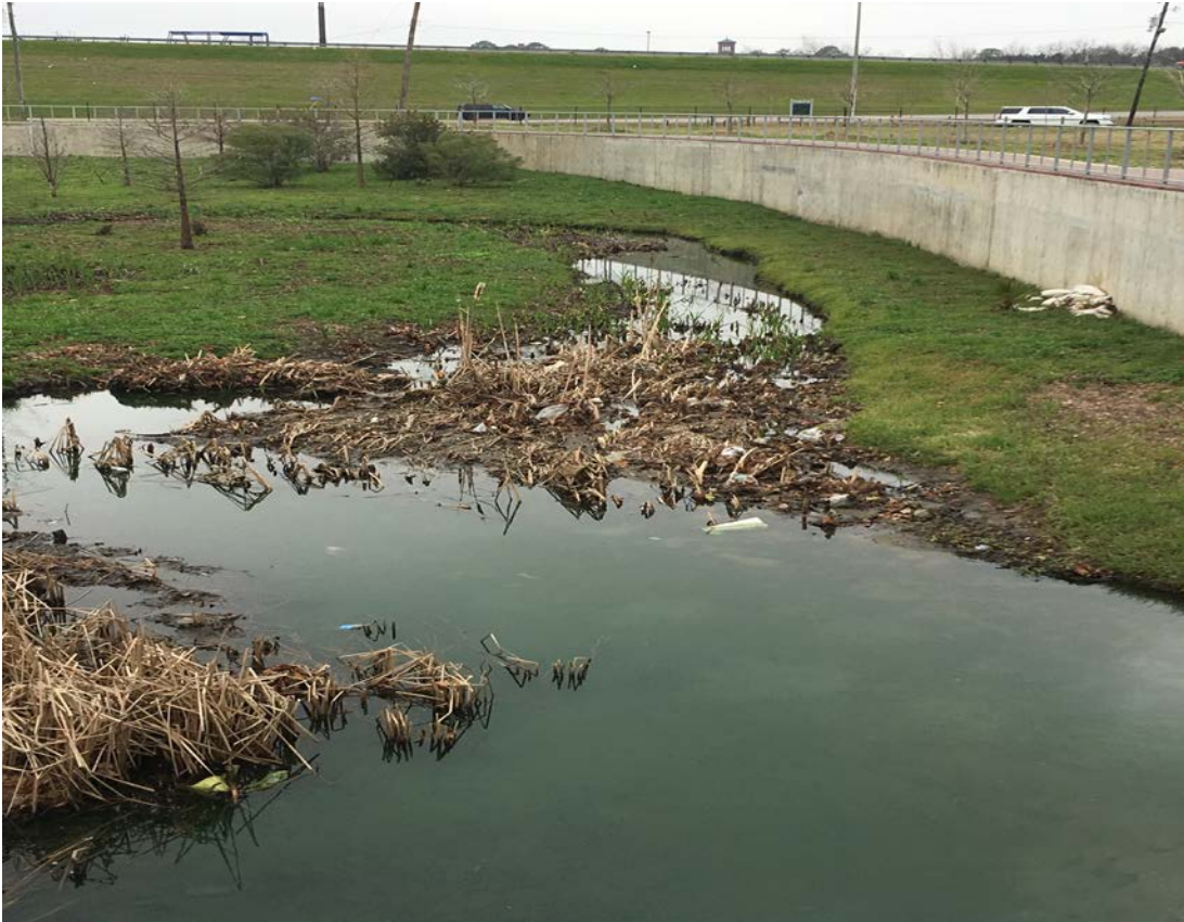
Figure 12 In-flow trash debris located in Fairview Environmental Park. Photo taken February 2, 2017.
